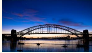
Sydney Harbour Bridge, Sydney, Australia
