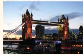
Tower Bridge, London, England
